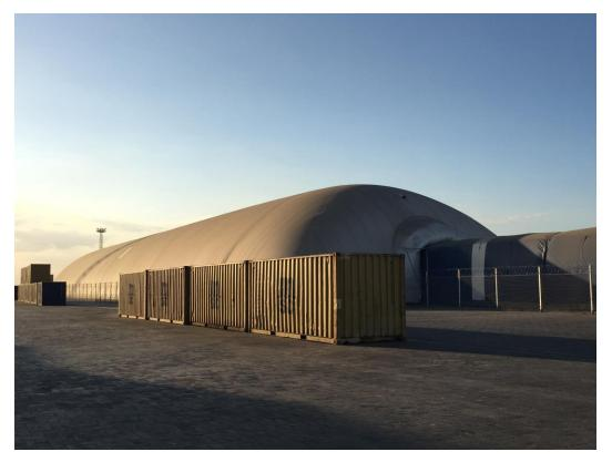
For large volumes of bulk exports, a dedicated finger terminal and storage area outside the existing port may be a solution. CDN has already provided an inflatable warehouse with a capacity of 12,000 t, with the advantage that it can be moved as port planning is finalised. CDN confirmed in December 2017 that they have acquired two additional inflatable warehouses with similar capacities, to be erected at Nacala port and Chipata. This is a planned marketing initiative rather than demand driven.
